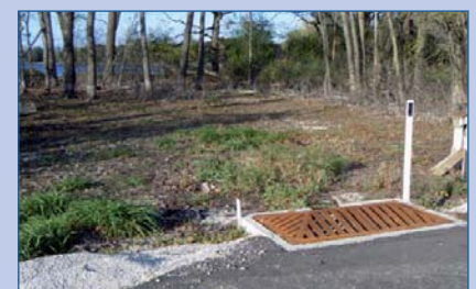
Water from lowlands enters outlet structure at Lower Lake Road
